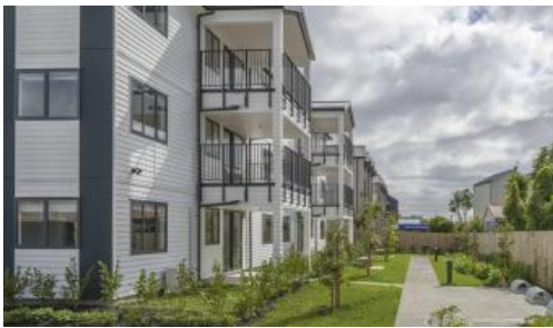
57 Henderson Valley Road, Henderson
